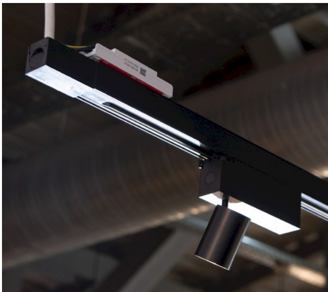
◀ Zumtobel installed 34 Supersystem II spotlights controlled via qualified Bluetooth mesh bmLINKs and a LITECOM controller
