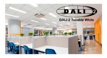
Commonly referred to as "tunable white", Tc allows control of the correlated colour temperature (CCT) along the black-body line, from warm white to cool white.
